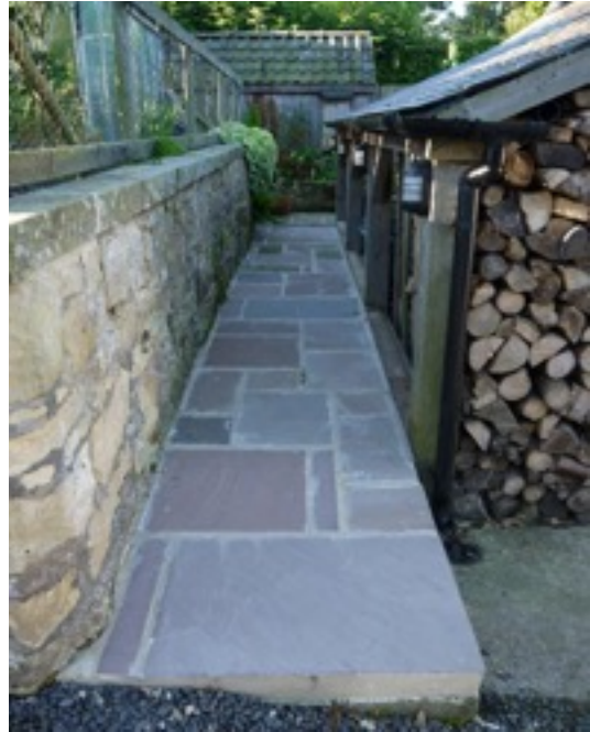
Figure 3 path to main entrance
