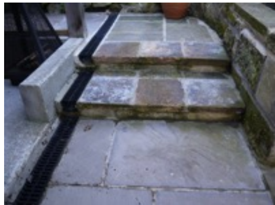
Figure 4 steps near main entrance
